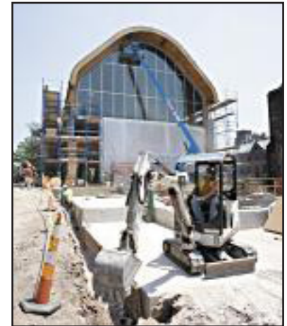
Kroon Hall, a New Haven project for Turner Construction Co., a nationwide contractor with offices in Milford, will showcase the latest developments in green building, combining cutting-edge technology and locally sourced materials.
